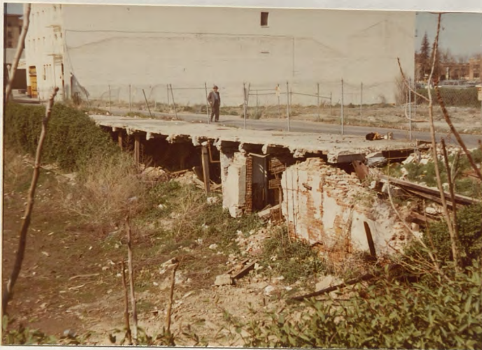
Part of the original ground level under downtown Sacramento near the corner of 10th & H Streets.
