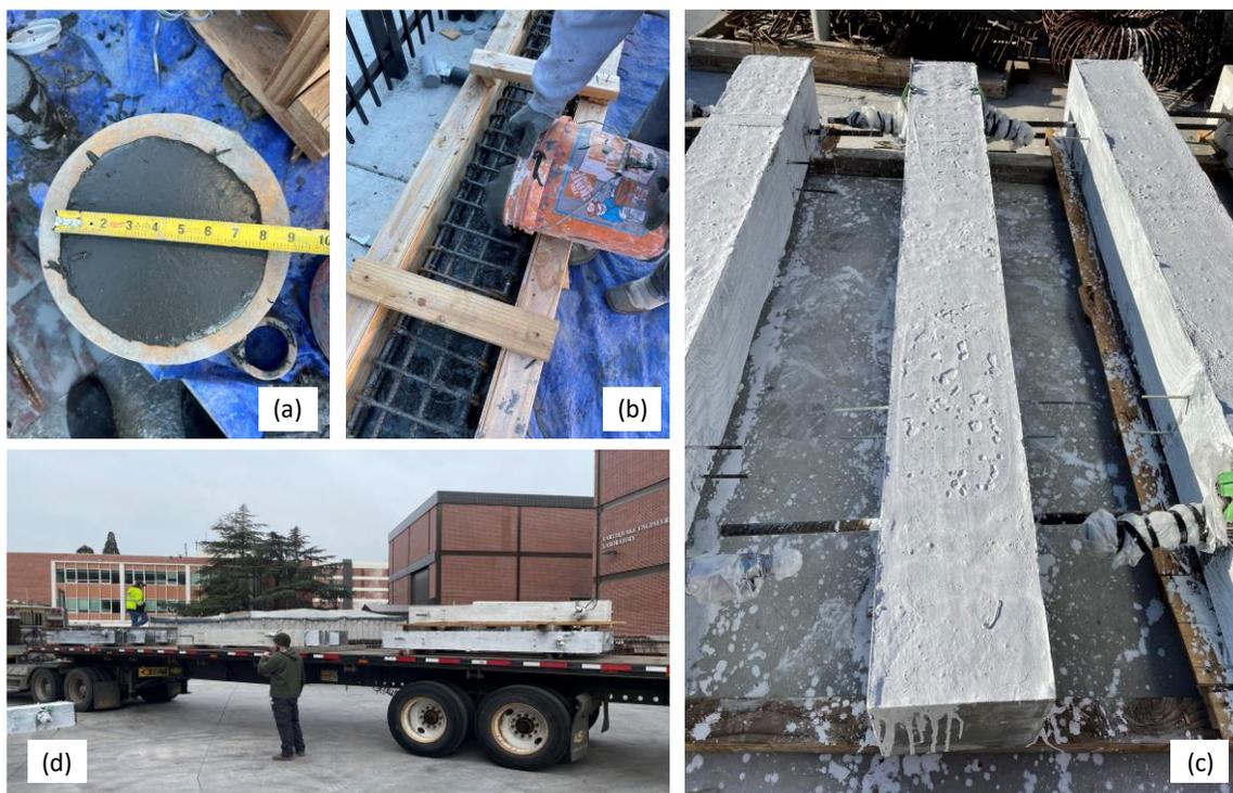
**Figure 3-12.** Photographs from columns construction: (a) flow test of one of one of the batches, (b) pouring UHPC into one of the columns, (c) completed columns with a coat of whitewash paint, and (d) loading the columns to a flatbed truck to be transported to the UC
