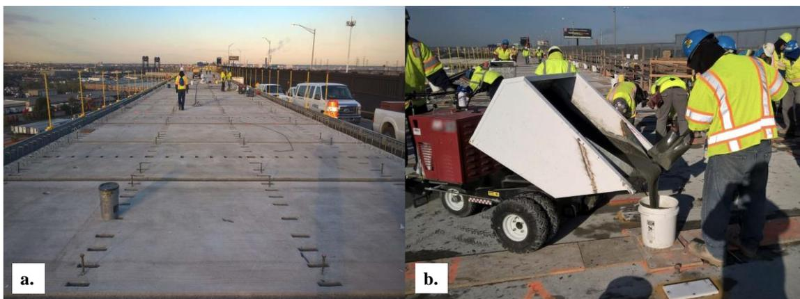
**Figure 3-1.** Most common application of UHPC in ABC: example from rehabilitation of Pulaski Skyway in New Jersey: (a) precast deck panels before furnishing UHPC; (b) casting of UHPC in the field joints [8]
