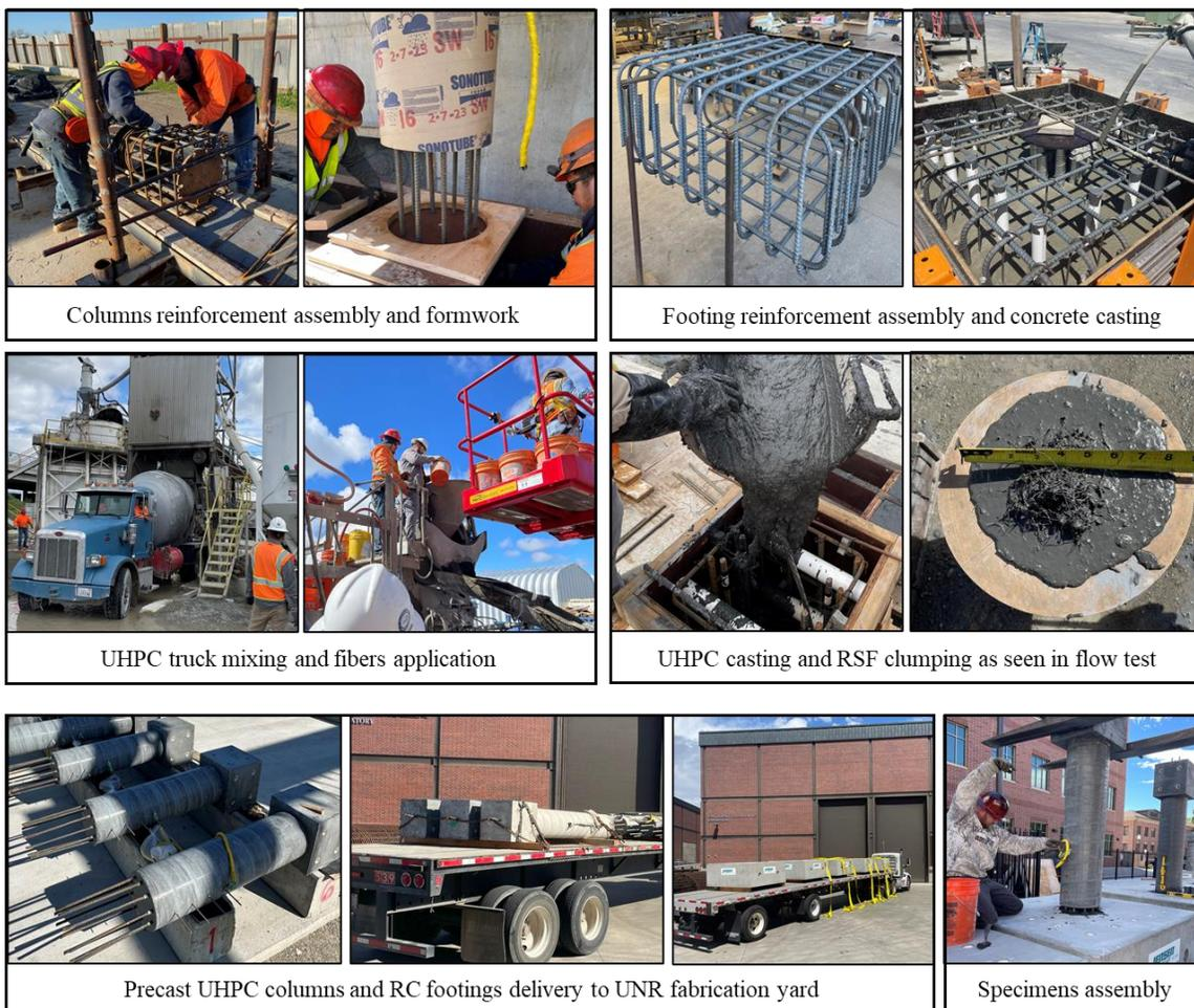
**Figure 5-3.** Fabrication, casting, and assembly of UHPC ABC columns
