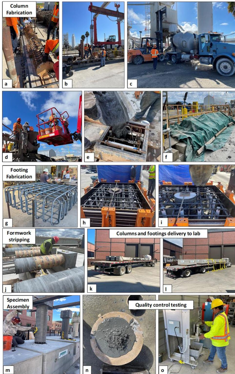
**Figure 4-4.** Catalog of photographs documenting the various construction phases of the test specimens
