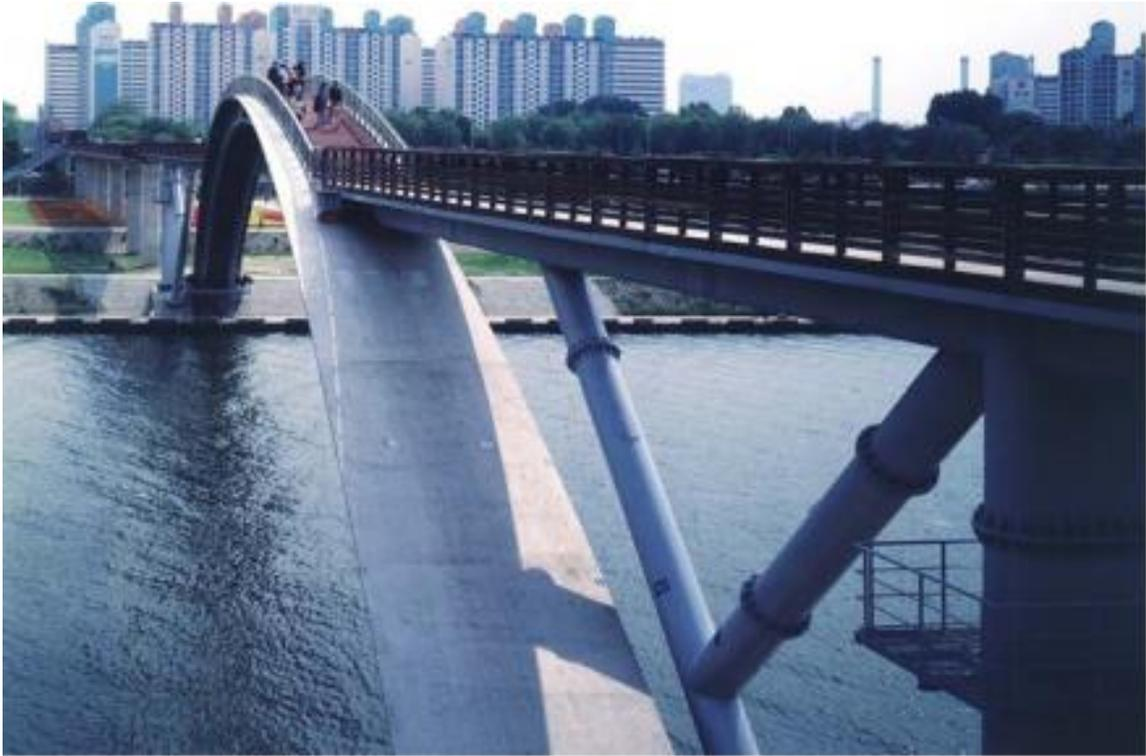
**Figure 1-1.** Completed Seonyu footbridge using Ductal UHPC [1]
