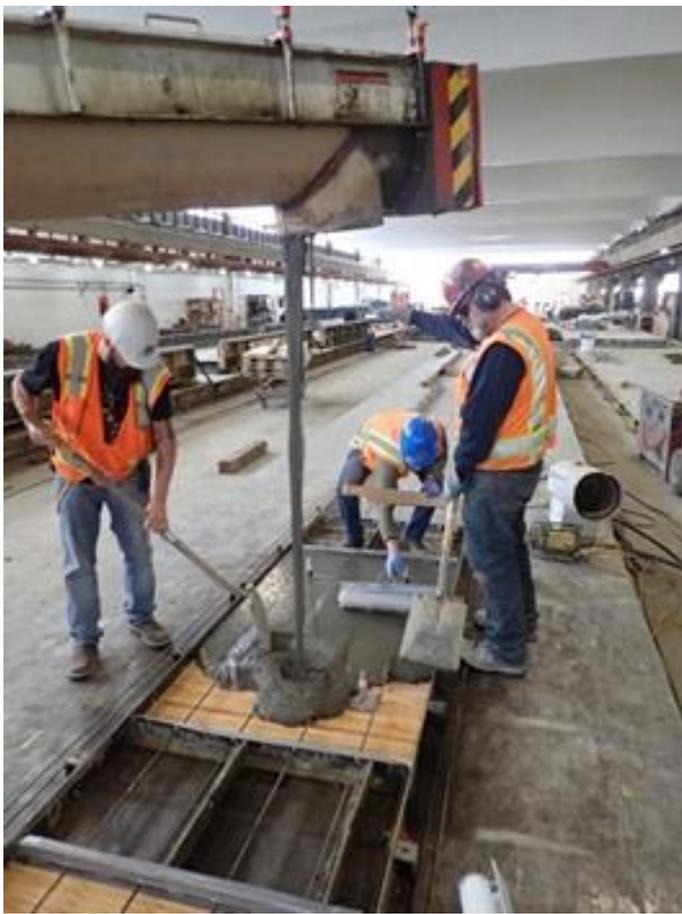
**Figure 1-2.** Placement of UHPC for precast applications [9]
