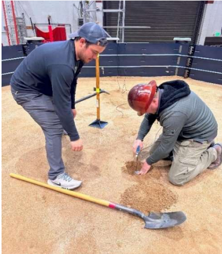
Figure 27: Installation of embedded accelerometers
