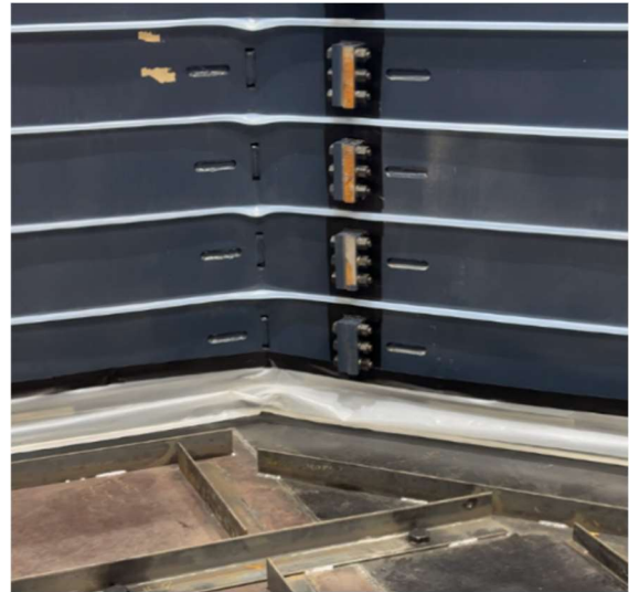
Figure 13: Plastic sheets sealing the gap
