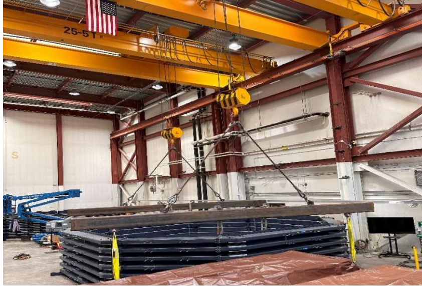
Figure 14: Hauling of soil box segment using double girder crane
