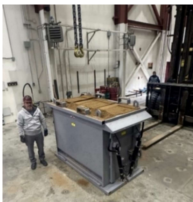
Figure 17: Hopper full of soil ready to be lifted
