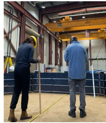
Figure 22: Measuring the level of compacted soil
