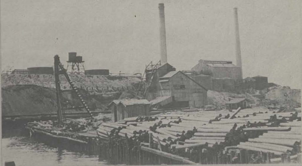
POWER PLANT - SANTA LUCIA
