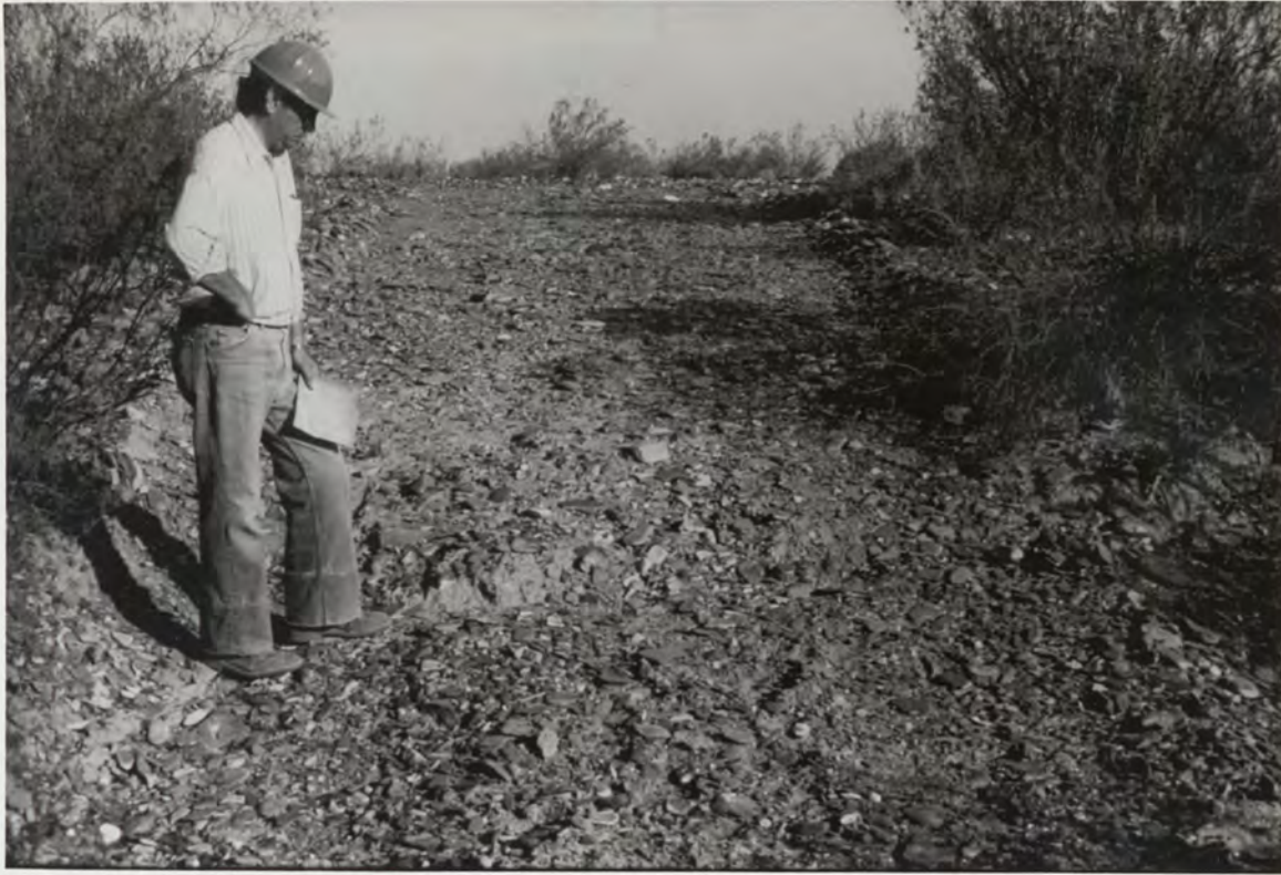
Figure 28. Photograph of displacement from the 1977 earthquake on an abandoned road across the Niquizanga fault zone. Displacement on this graben was about 4 inches (10 cm) on each side of the graben, in an opposite sense. Trench 10 was placed in the roadbed (see Figure 29 and log of Trench 10).
