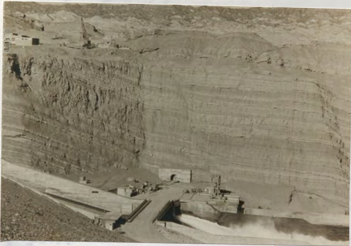
Figure 19. Photograph of normal fault graben formation in the north wall of the spillway of the Dique de Ullun.
