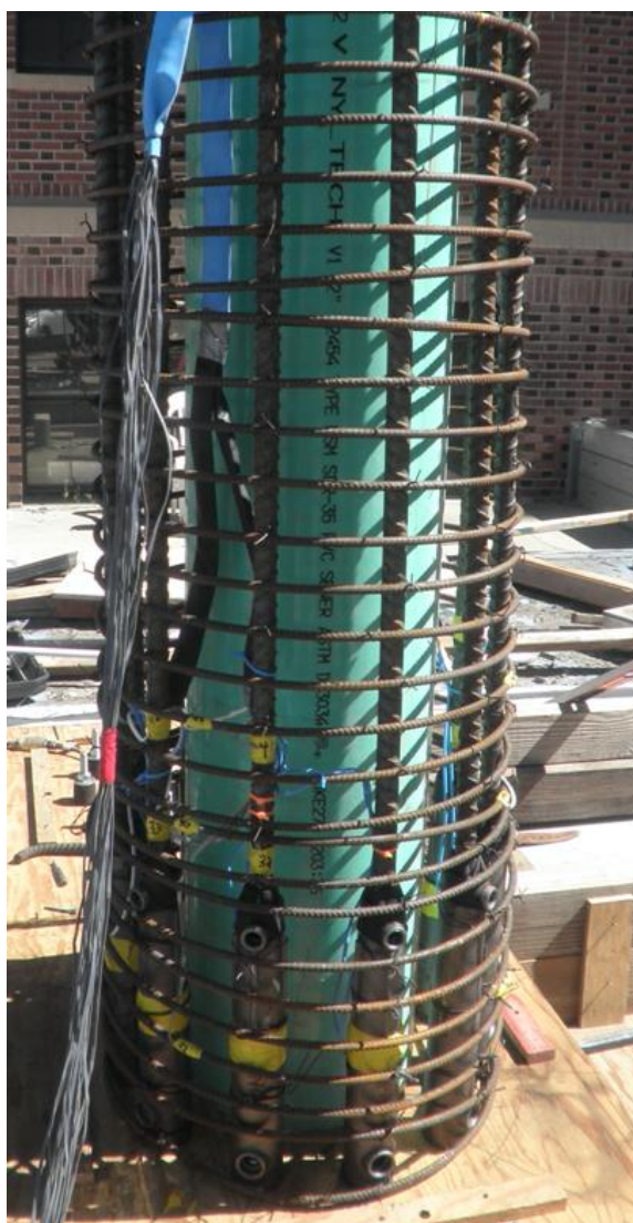
Figure 3-75 GCNP column cage on platform with PVC form in the center
