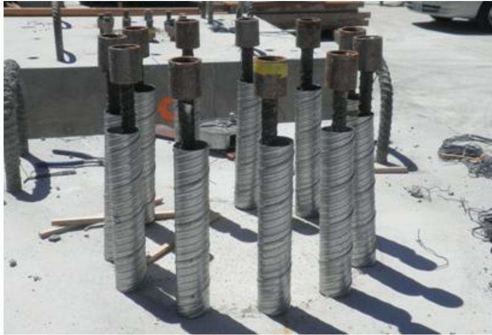
Figure 3-48 HCPP footing dowels and placement of corrugated ducts for pedestal
