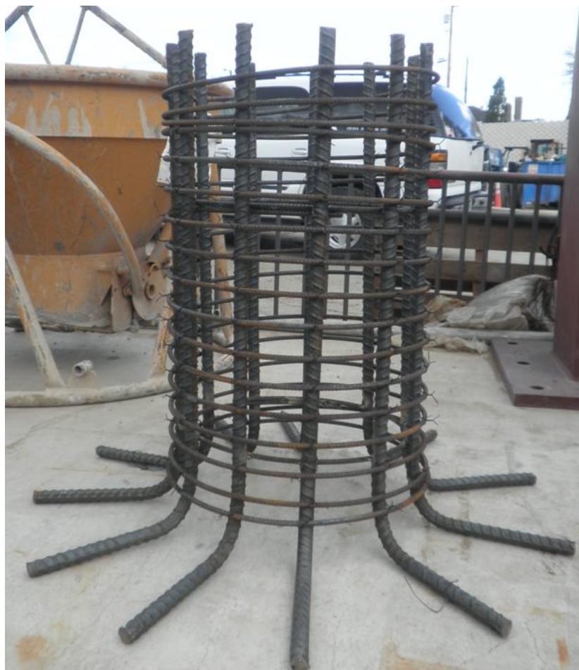
Figure 3-66 GCNP footing dowel reinforcement cage
