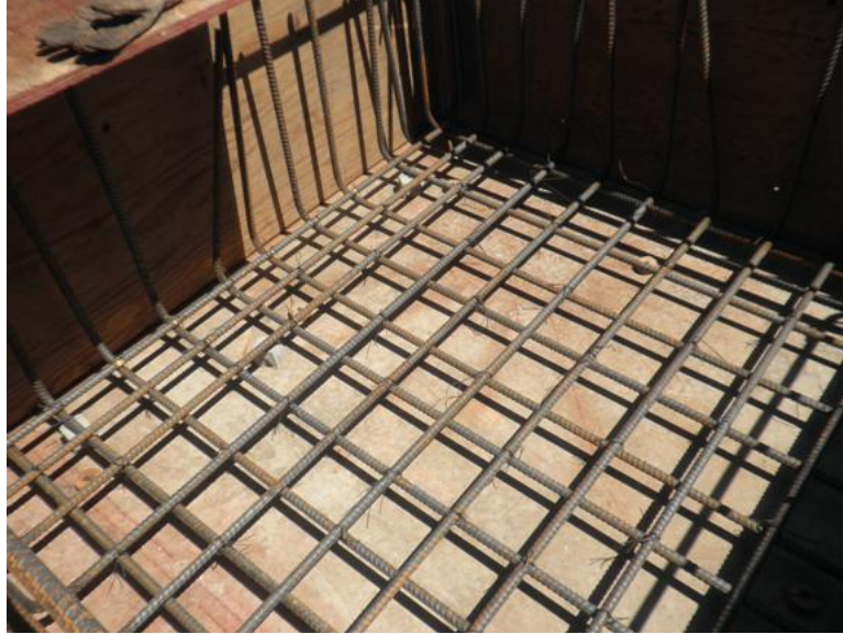
Figure 3-6 Bottom steel in footing form
