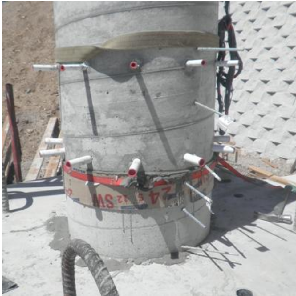
Figure 3-88 Placement of the GCPP column shell
