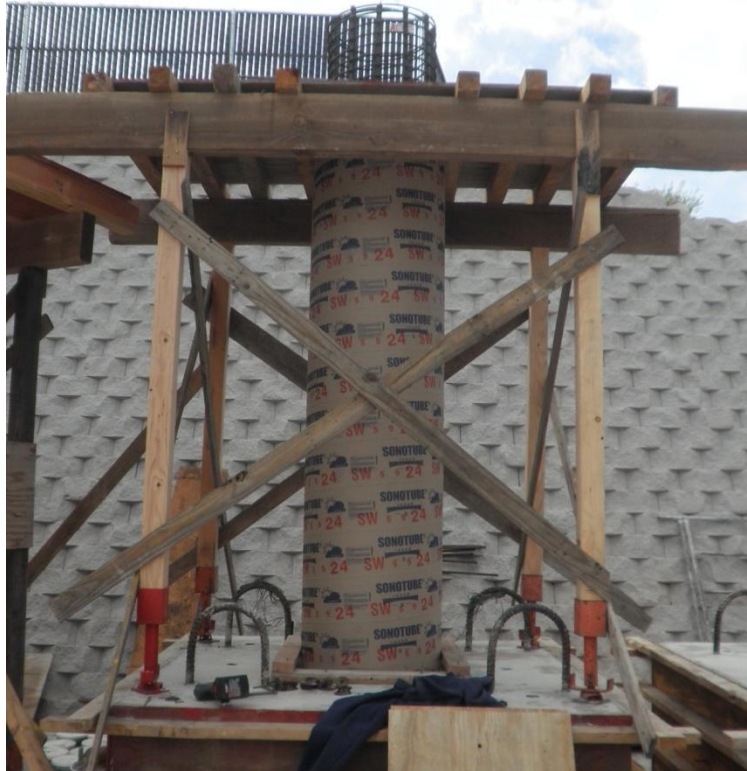
Figure 3-8 Form-work for column ready for head construction
