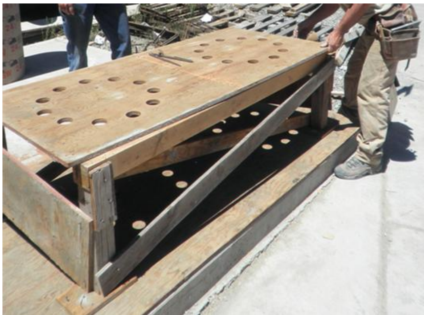
Figure 3-24 Prepared form-work for HC column base segment
