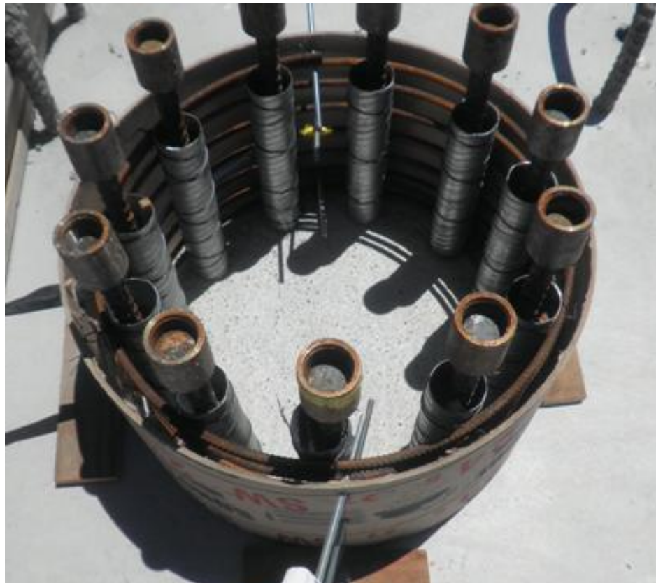
Figure 3-49 Pedestal reinforcement and form-work
