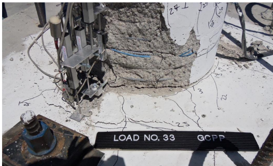
(a) Footing damage on west face during first push cycle
