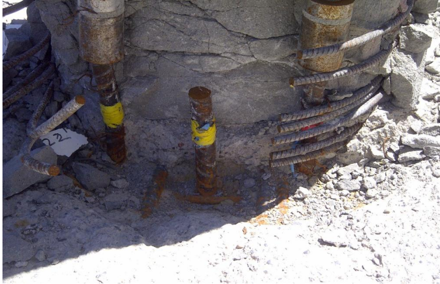
Figure 4-45 Removal of concrete from plastic hinge and footing
