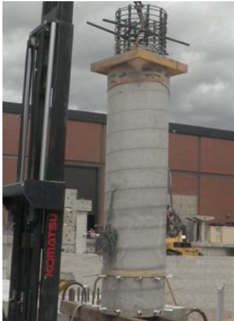
Figure 3-77 Complete GCNP column shell
