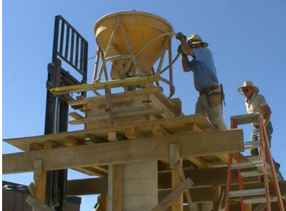
Figure 3-46 Cast SCC in column core
