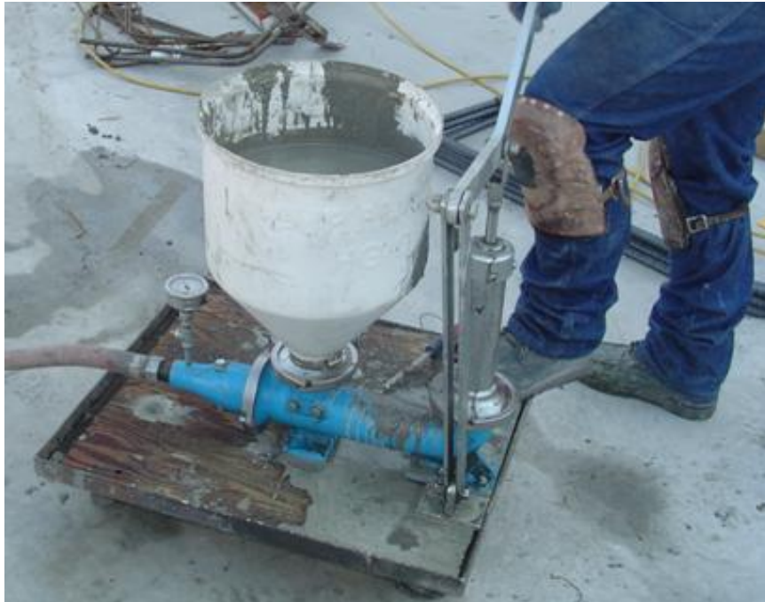
Figure 3-36 Grout ready for pumping
