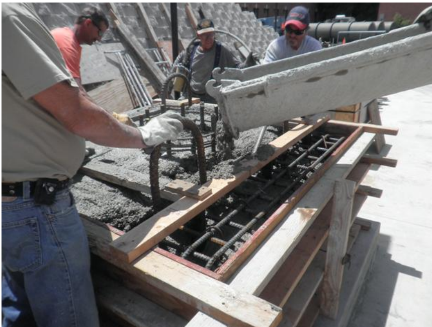
Figure 3-68 GCNP footing casting concrete
