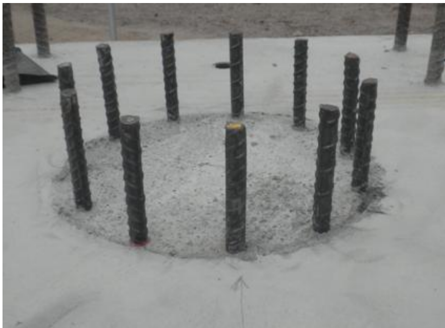
Figure 3-79 GCNP footing dowel bars after cleaning
