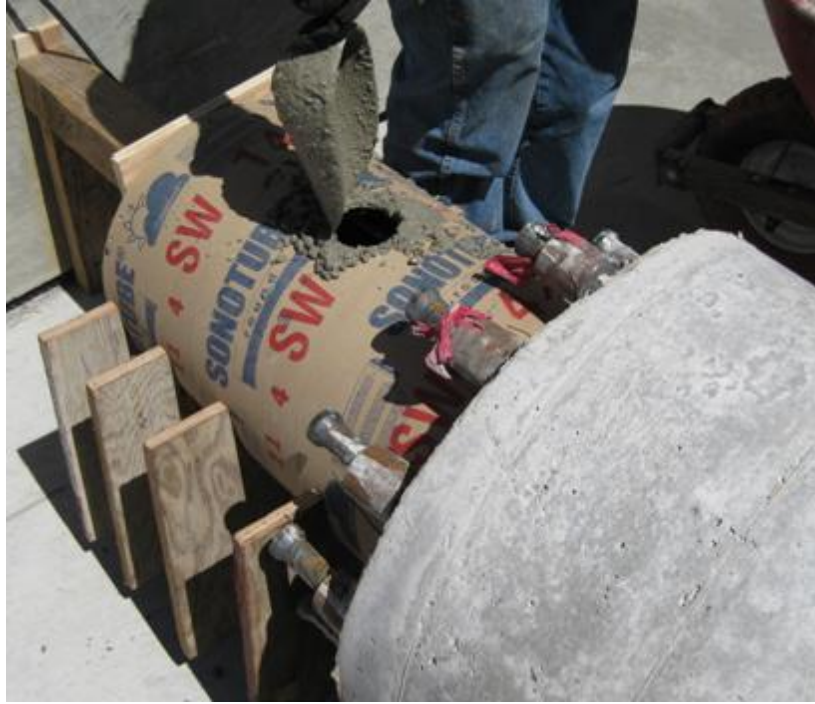
Figure 3-52 Repair form-work and casting of new concrete
