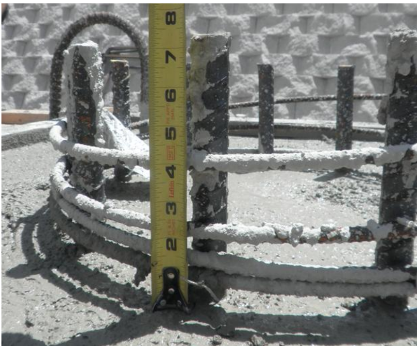
Figure 3-69 Measurement of GCNP footing dowel
