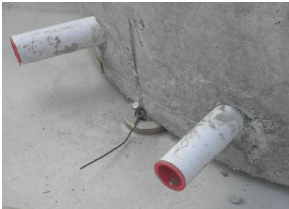
Figure 3-81 Steel shim between column shell and footing
