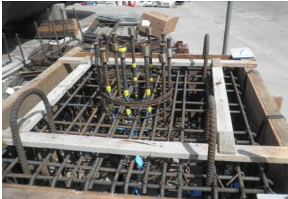
Figure 3-47 HCPP footing reinforcement and form-work
