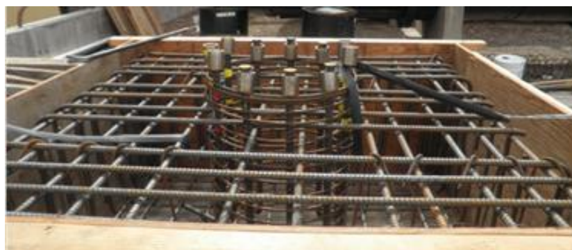
Figure 3-22 HCNP footing reinforcement and form-work prior to casting concrete
