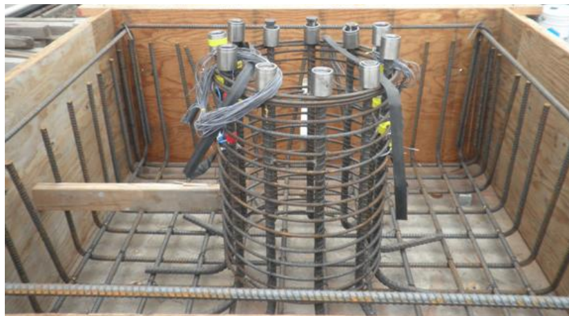
Figure 3-21 Placement of HCNP footing column cage
