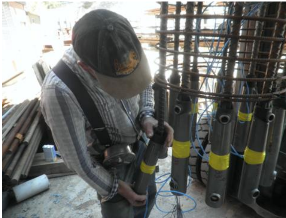
Figure 3-71 Installation of NMB couplers on GCNP column cage
