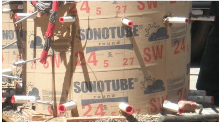
Figure 3-76 Grout ports protruding through form
