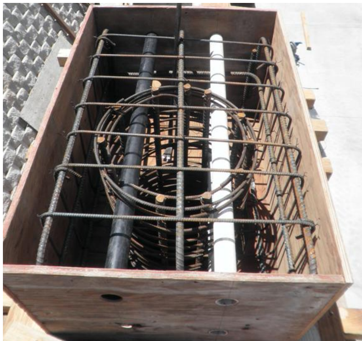
Figure 3-9 CIP column head formwork and reinforcement
