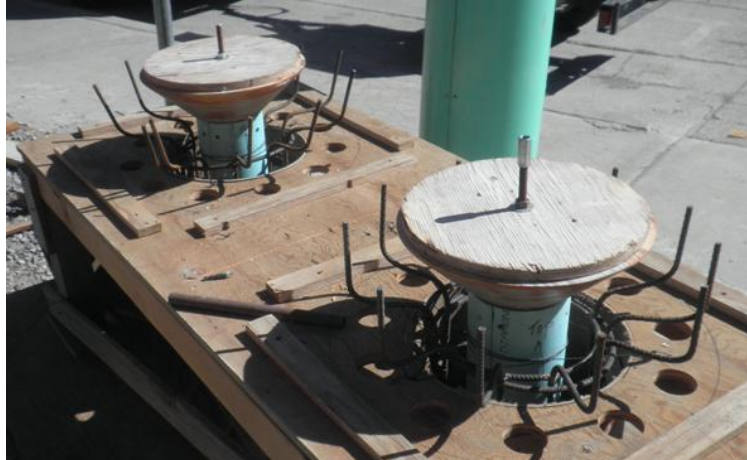
Figure 3-25 Construction of column cage base segment
