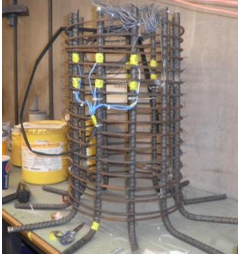
Figure 3-90 Wiring of GCNP footing cage
