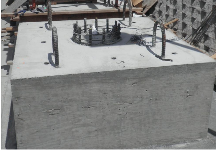
Figure 3-70 GCNP footing after removal of formwork
