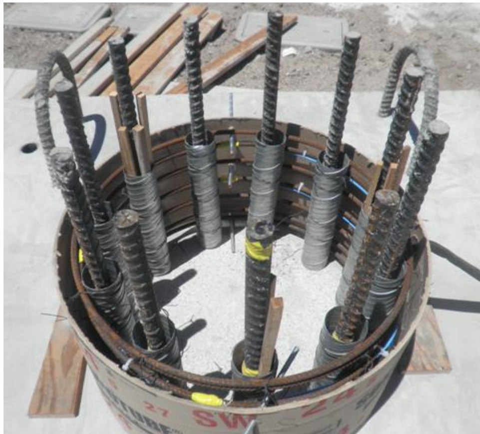
Figure 3-85 GCPP pedestal formwork and reinforcement
