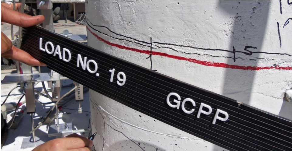
(a) Concentrated crack ( \approx 0.08 in [2 mm]) at pedestal-column joint during second push cycle
