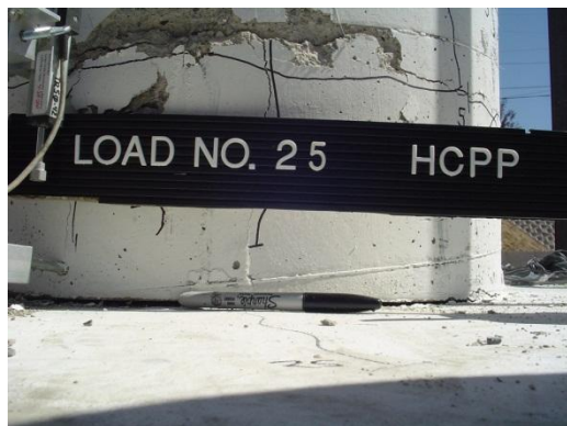
(a) Pedestal-footing joint during first push cycle (West face)
