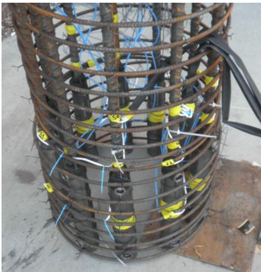
Figure 3-93 GCNP column cage instrumentation
