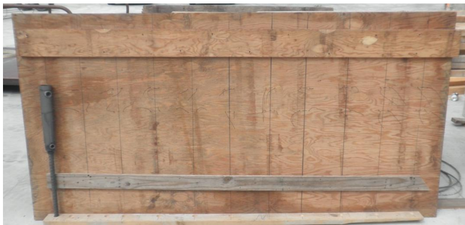
Figure 2-13 Support frame for construction of grouted coupler specimens
