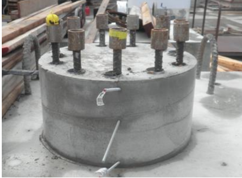
Figure 3-50 HCPP pedestal after casting concrete
