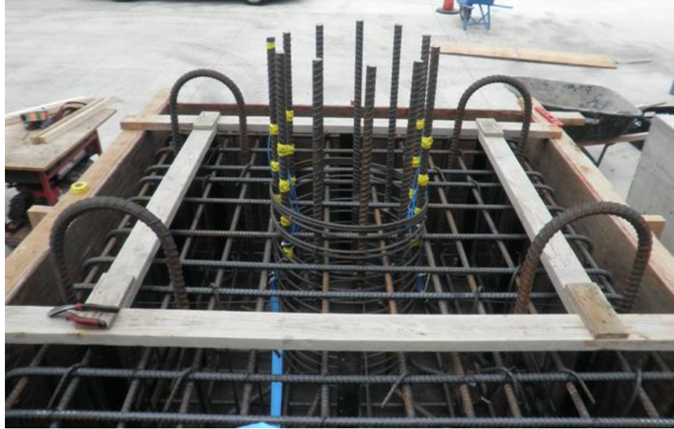
Figure 3-84 GCPP footing formwork and reinforcement
