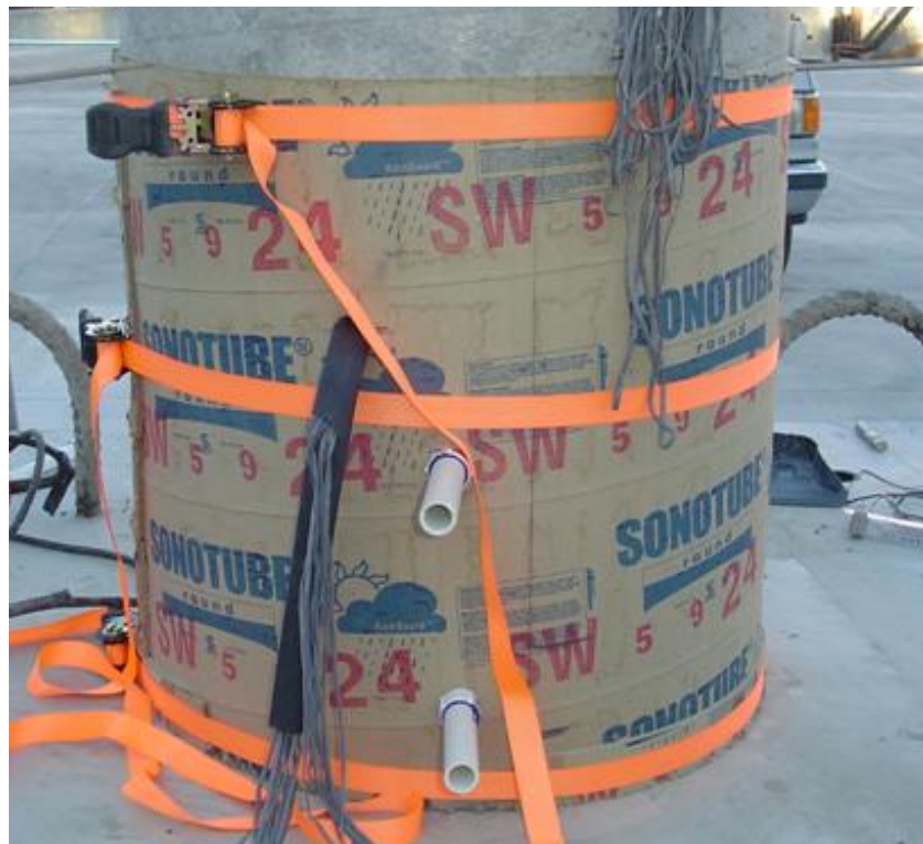
Figure 3-35 Connection region ready for closure grouting
