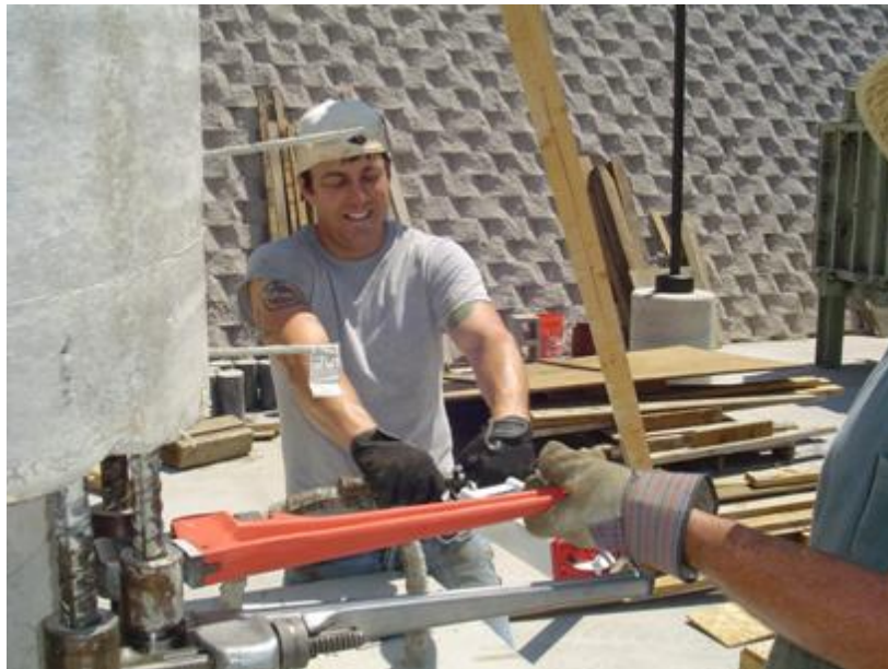
Figure 3-33 Torqueing HRC couplers
