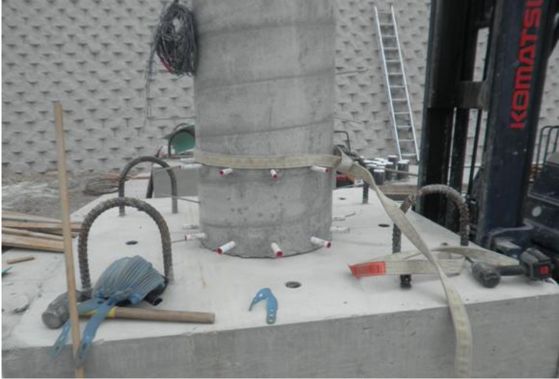
Figure 3-80 GCNP column shell after placement on footing dowels
