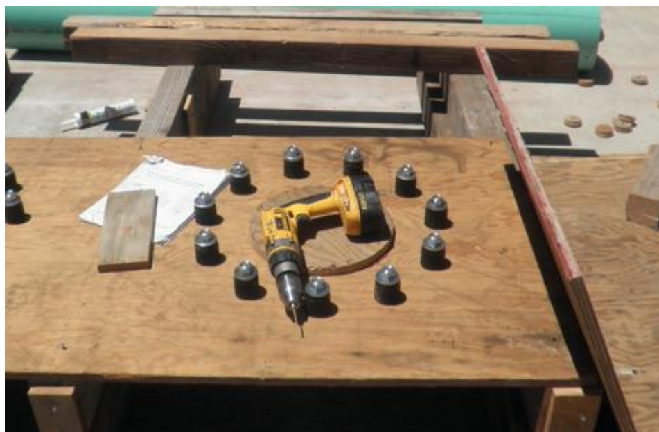
Figure 3-73 GCNP column shell platform with NMB Sleeve Setters
