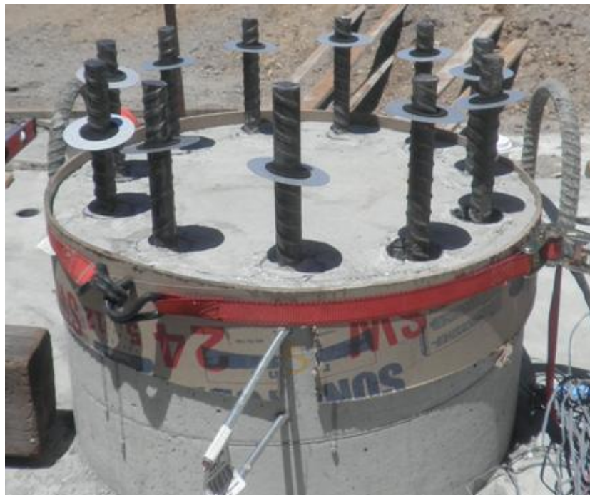
Figure 3-87 Temporary grout form and grout washers
