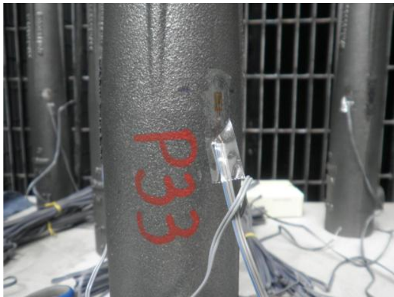
Figure 3-91 Strain gage installation on NMB couplers
