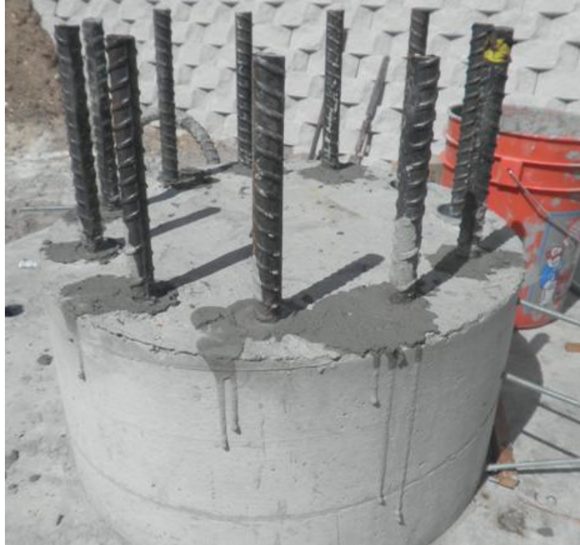
Figure 3-86 GCPP pedestal ducts after grouting and cleaning dowels
