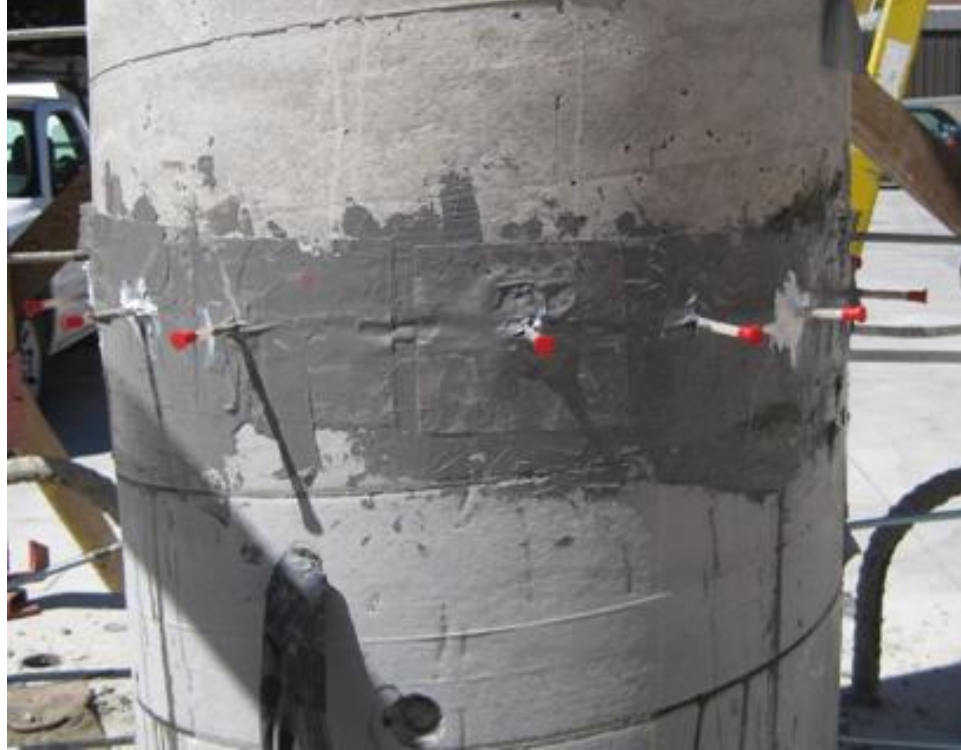
Figure 3-40 Void region prepared for epoxy injection
