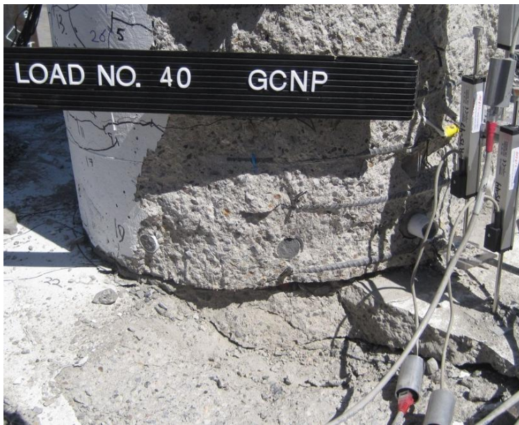
(a) Footing damage on west face during first push cycle
