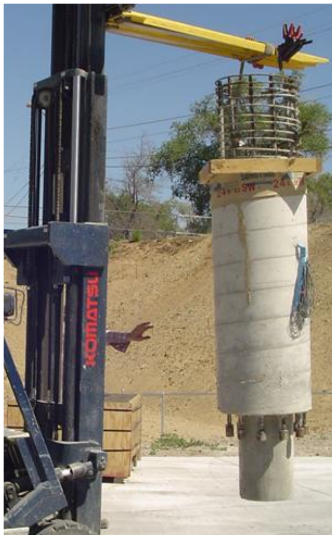
Figure 3-28 HCNP column shell after removal of formwork
