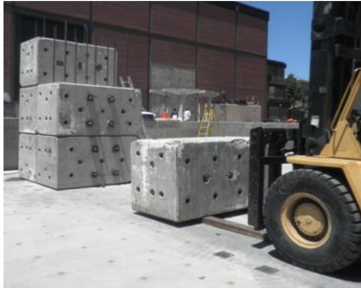
Figure 3-100 Construction of reaction pylon
