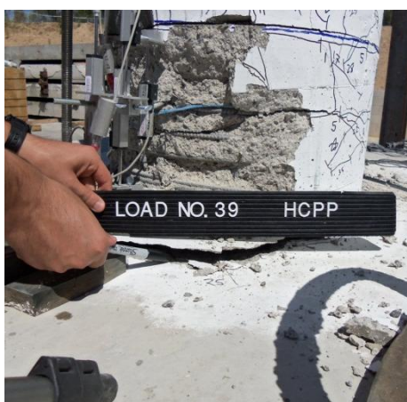
(a) Pedestal-footing joint during second push cycle (West face)
