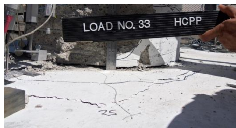
(a) Pedestal-footing joint during first push cycle (West face)
