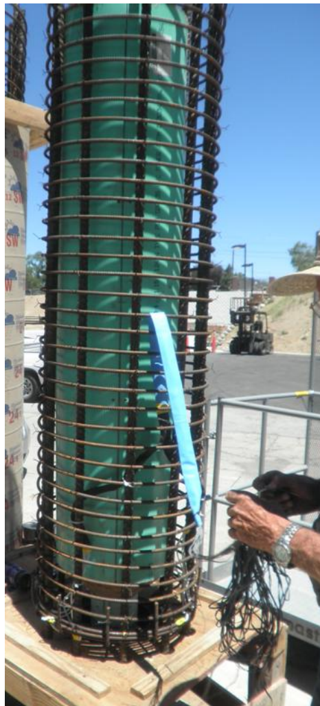
Figure 3-26 Column cages and internal PVC form
