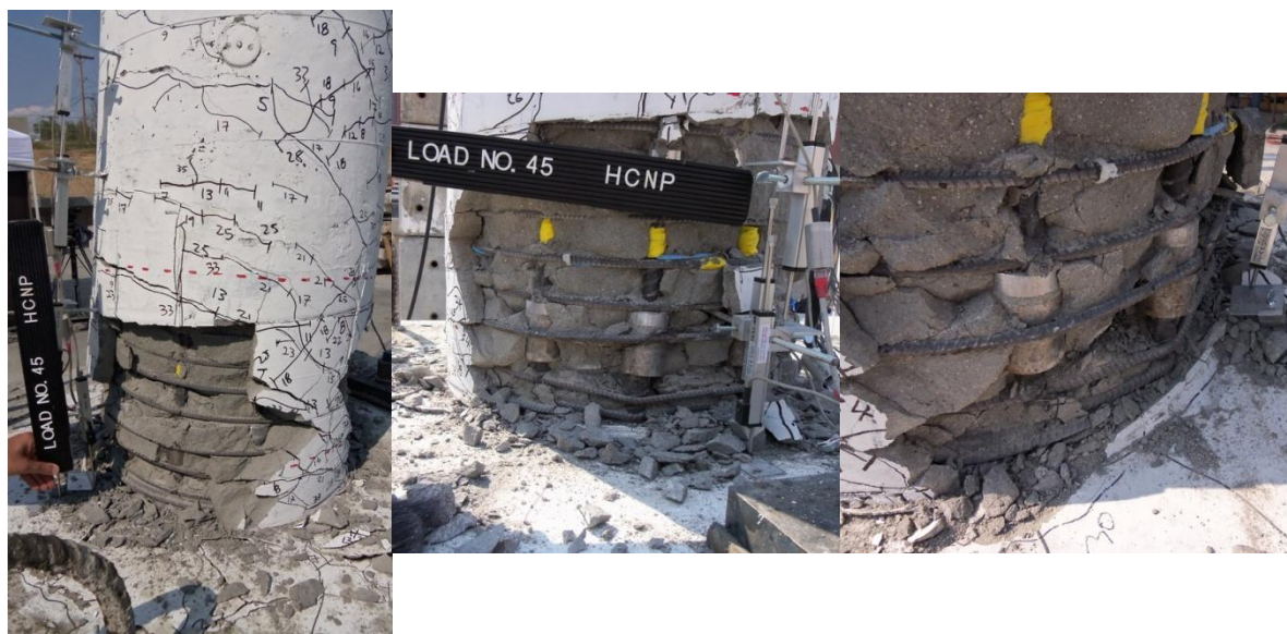
(a) South-west face (b) East face (c) Close-up on east face
