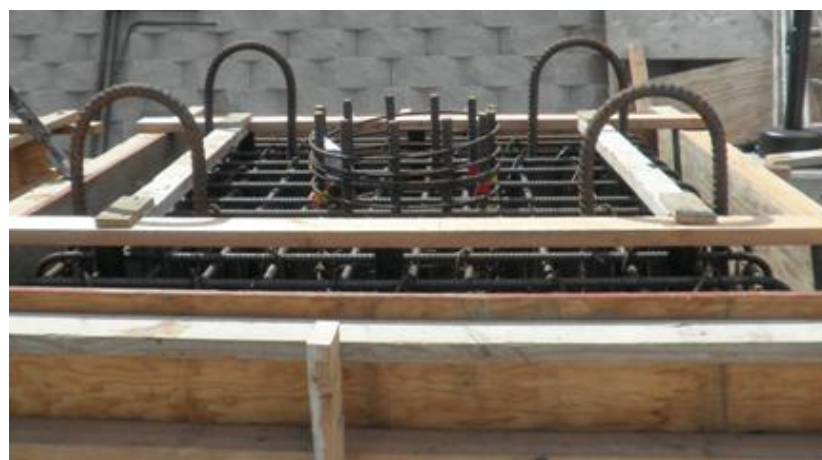
Figure 3-67 GCNP completed footing form and reinforcement
