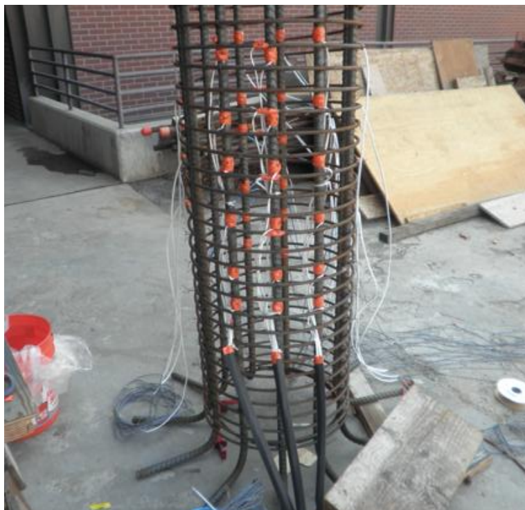
Figure 3-12 Instrumented cast-in-place column cage
