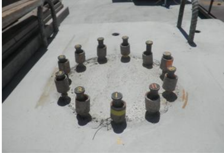
Figure 3-23 Footing after casting showing HRC headed dowels
