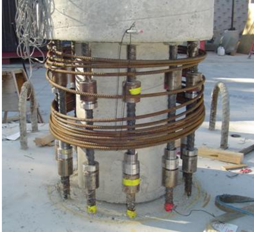
Figure 3-30 Initial setting of HCNP column shell
