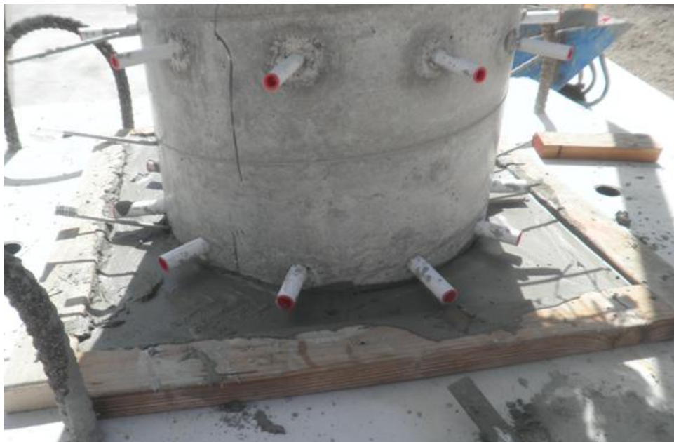
Figure 3-83 Grout after placement
