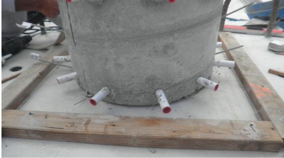
Figure 3-82 Temporary formwork for grouting column shell-to-footing interface
