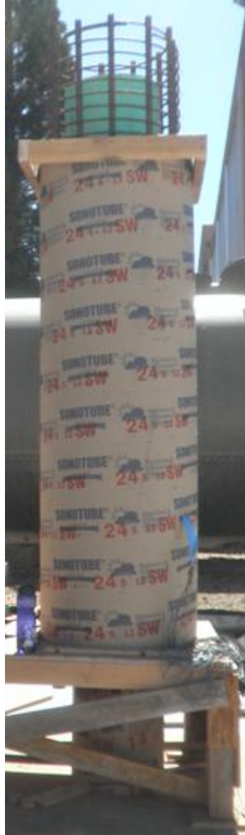
Figure 3-27 HCNP column sell ready for casting concrete
