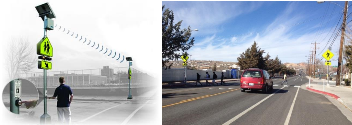
Figure 43 Currently Installed RRFB in Sutro Street, Reno, NV
