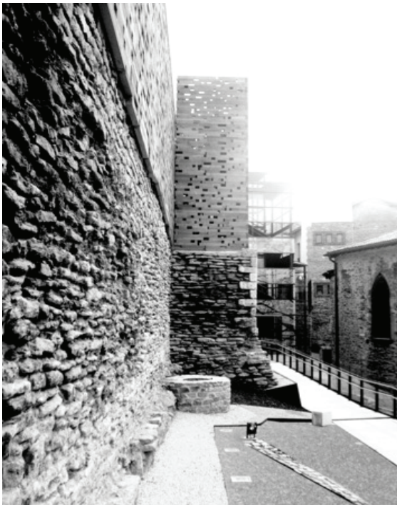
Figure 6.6 Wall panels and access ramps as seen from the south.
