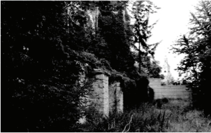
Figure 6.4 Previous state of the space adjacent to the walls.
