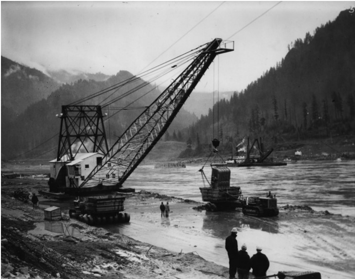
Figure 4-9. “Crane Dredging at Bonneville Construction Site, 1935?”
