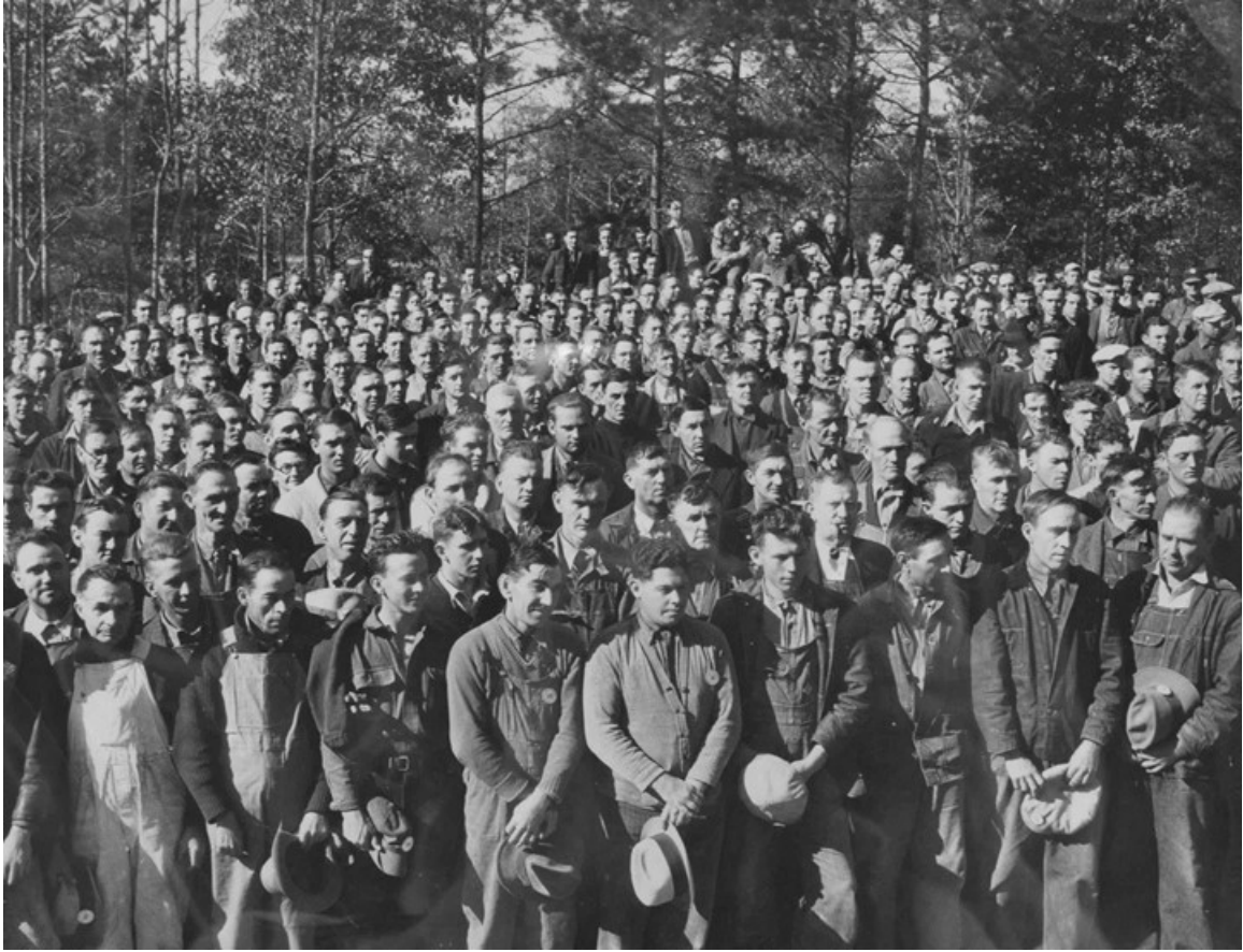
Figure 6-6. Workers at Norris Dam construction camp.
