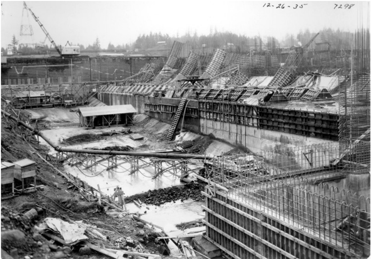
Figure 4-10. Construction at Bonneville.
