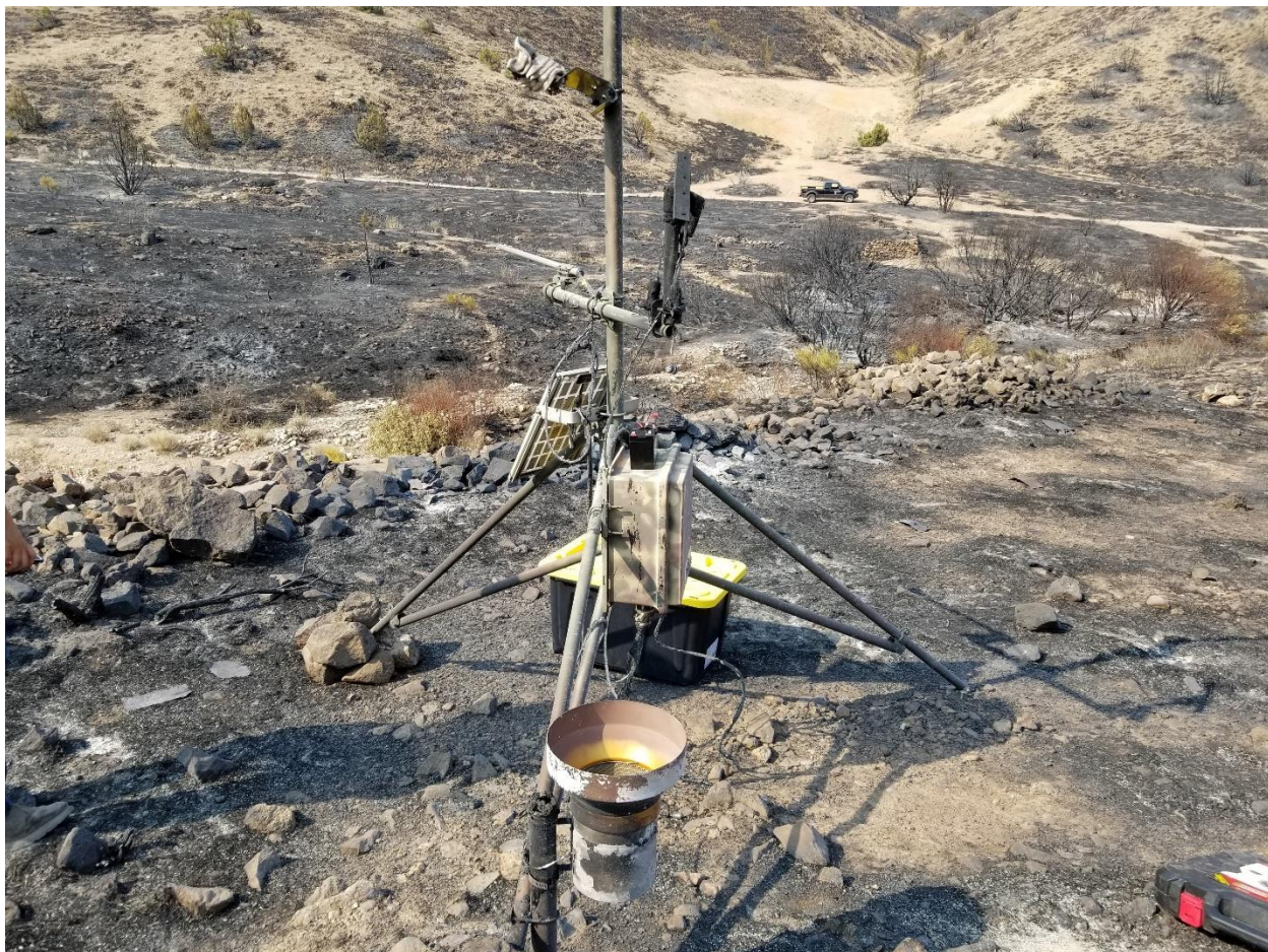
Figure 8: Picture of the MET Station after being destroyed in the Perry Fire in July 2018.
